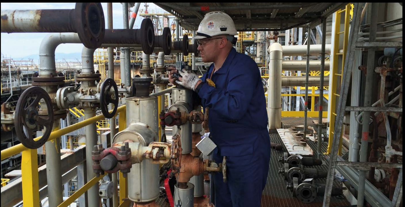
Below: Destec Inspector onsite at Milazzo Refinery.
